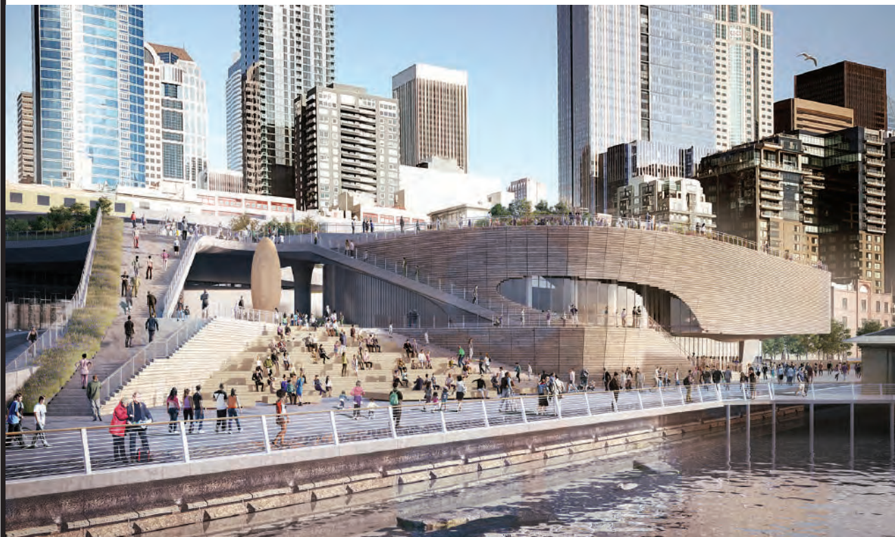
LMN Architects ( No. 37 ) is providing planning, architecture and design services on the Seattle Aquarium's new Ocean Pavilion. The building, with 50,000 sq ft of exhibition space, is designed to be all-electric and targets a 95% operational carbon reduction compared to similarly-sized aquariums. It will also filter and recycle 96% of its seawater. The project team is seeking both Living Building Challenge Petal Certification for energy, water, beauty, equity and place, and LEED Gold certification—the latter a requirement for all city-owned buildings.
