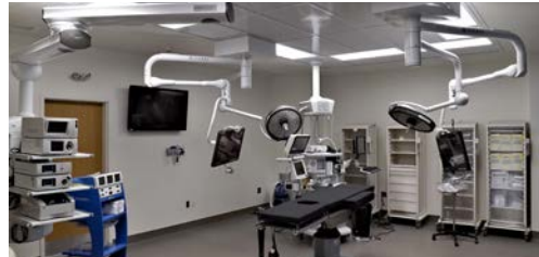
GRAY'S WOODS SURGERY CENTER & PARKING DECK GEISINGER HEALTH SYSTEM $35.1M 163,960 SF
