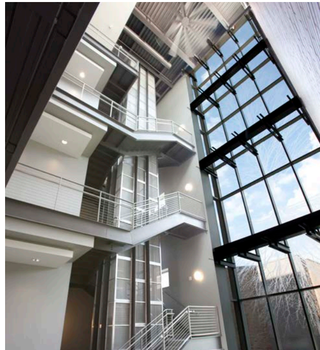
STEPS BUILDING LEHIGH UNIVERSITY $78.5M 130,000 SF
