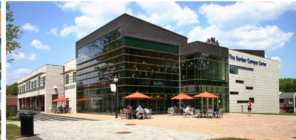
KANBAR CAMPUS CENTER AND PARKING GARAGE PHILADELPHIA UNIVERSITY $50.9M 155,000 SF
