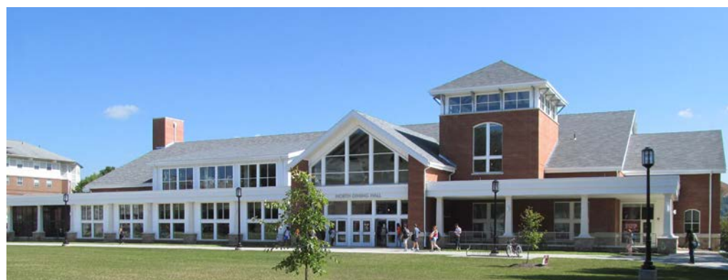
NORTH HALL DINING FACILITY INDIANA UNIVERSITY OF PENNSYLVANIA $22.1M 31,300 SF
