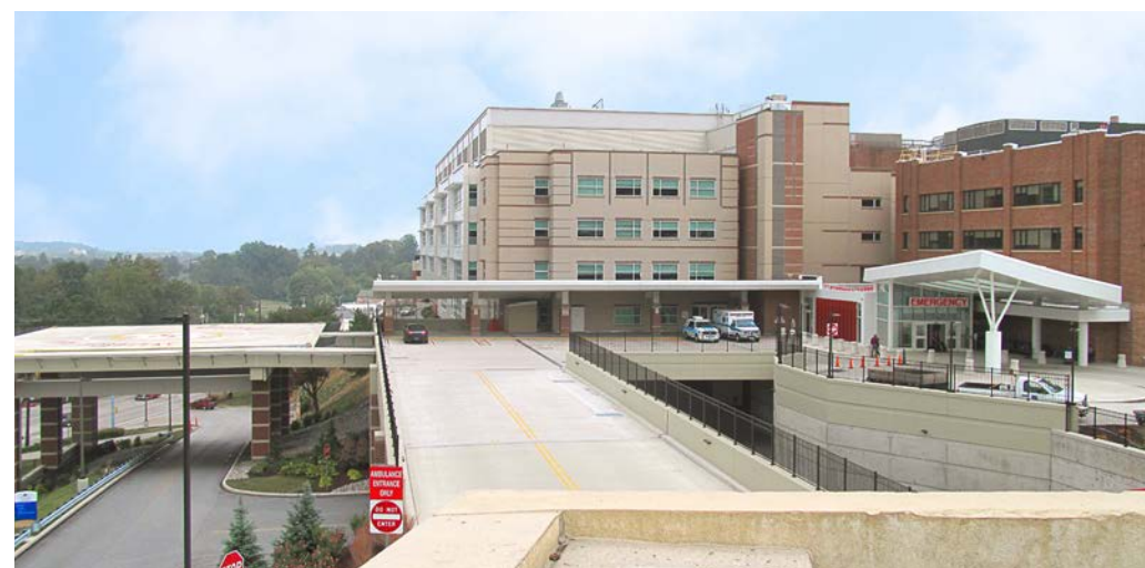
YORK HOSPITAL E.D. EXPANSION WELLSPAN HEALTH
