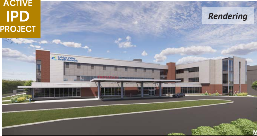
MUHLENBERG ED EXPANSION LVHN | JEFFERSON HEALTH
